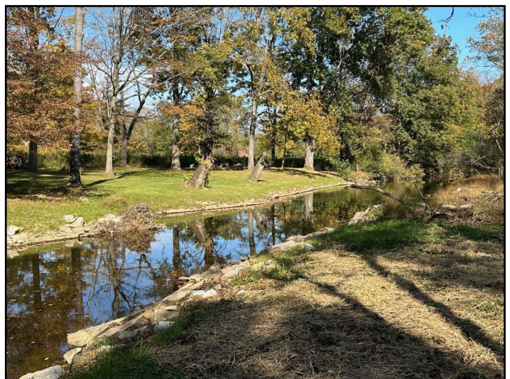
A modified mudsill structure installed along a 750 foot section of Fourmile Run in Cook Township.
